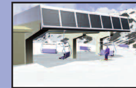
Ski lift passenger approaches dismount area at lift travelling speed. Safe acceleration/ deceleration and safe maximum speed allows travel in between stations to be smooth, constant and below a maximum speed.
